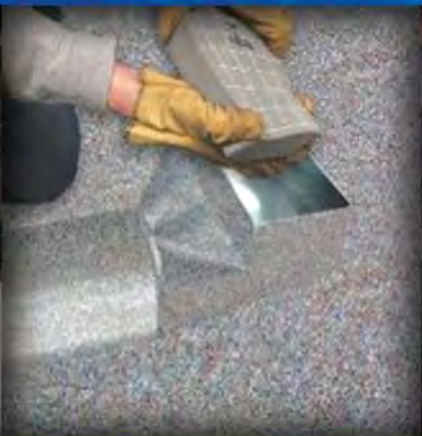
Wall registers are covered in order for air to escape only through leaks
