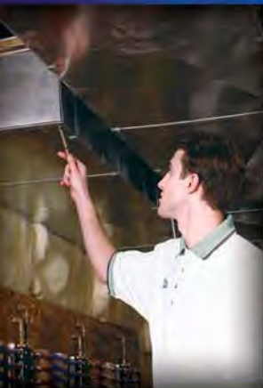
Aeroseal technician conducts initial diagnosis by analyzing airflow
